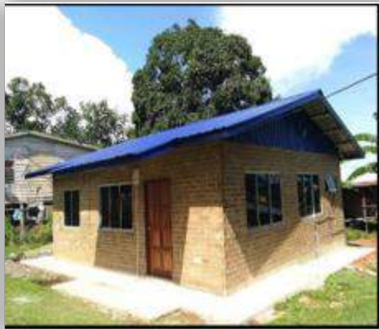
Photo 8: Ground floor plan and photo of Tawau residential building using ICEB construction (credit: Makiga Company/ Kampala)
